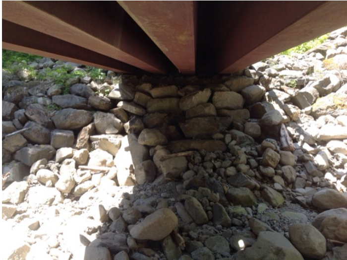
Right Bank Abutment when facing downstream
