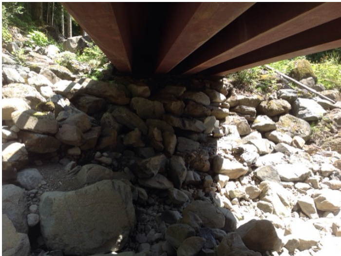
Left Bank Abutment when facing downstream
